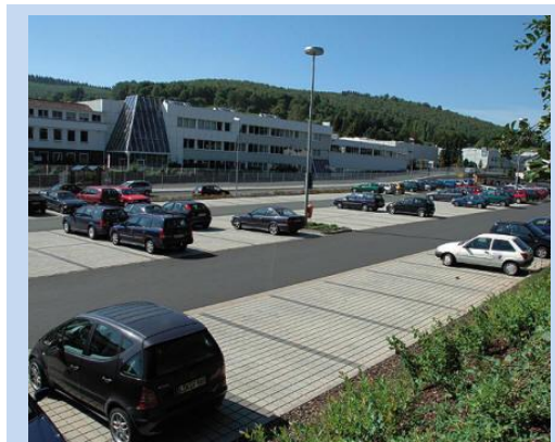
Illustration of porous pavement used in a parking lot to allow stormwater to pass through the pavement.
